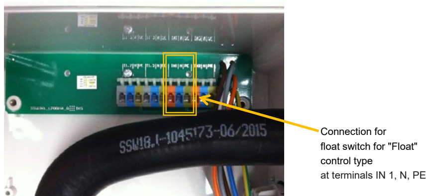
Figure 21: Float connection for clear water pump in K-Pilot 18.3/18.4 controller
