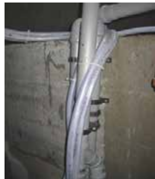
Hoses routed upwards on the lifters
