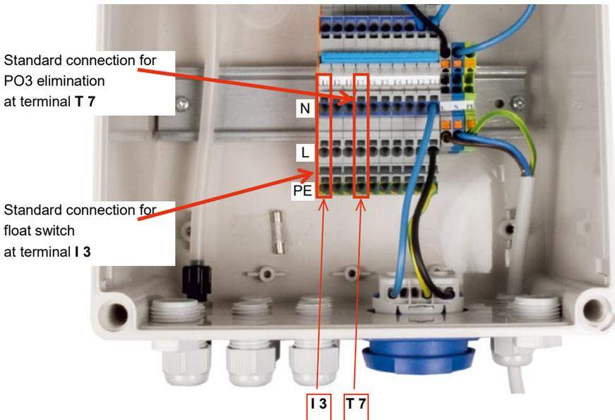
Figure 26: K-Pilot 9.7 controller – phosphate precipitation connection
