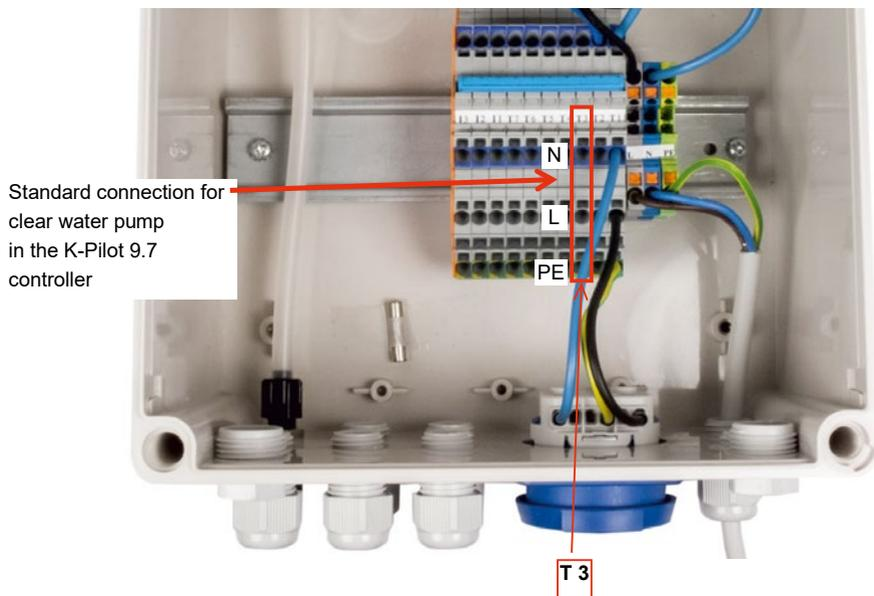
Figure 17: K-Pilot 9.7 controller – clear water pump connection
